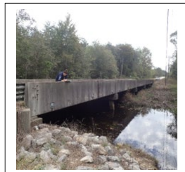
View of Bridge
