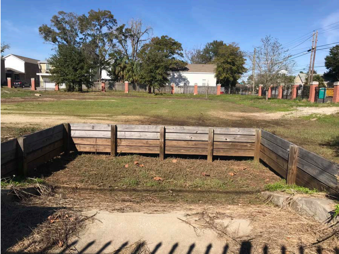
ECUA Dry Detention Pond at the lift station on Government Street and DeVillers
