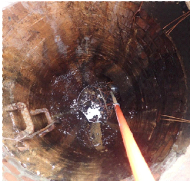
Figure 5- Deep stormwater outfall showing groundwater seeps entering through the joints between bricks (seen as darker streaks)
