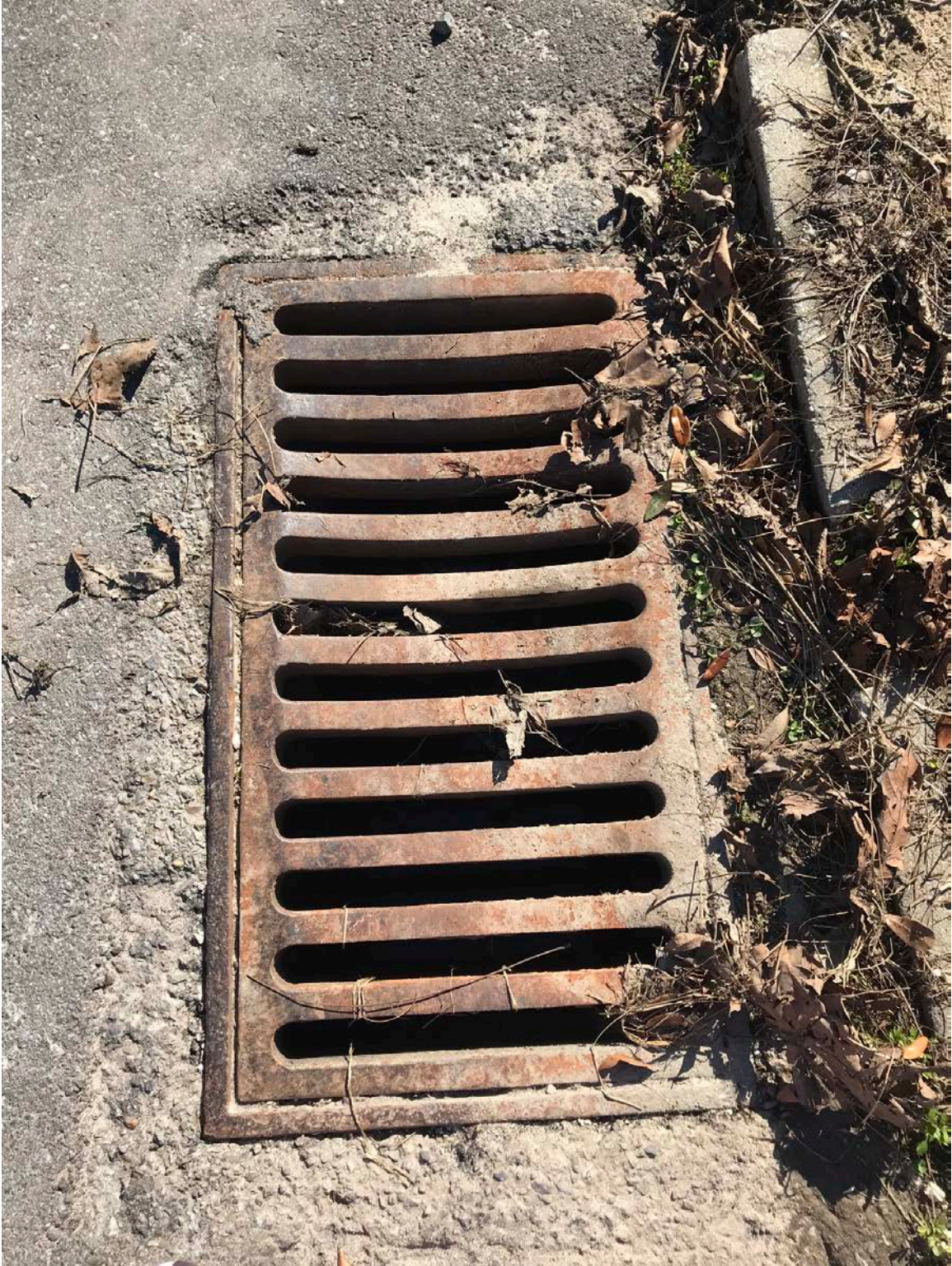
Small Stormwater Grate Inlet on the corner of Government and DeVillers Streets.
