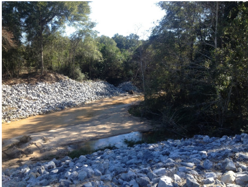
View of the 'stabilized' buried creek feeding into Ferry Creek Marina. Note the rip rap lining the creek bank. No native plantings for habitat were included for this stabilization project.
